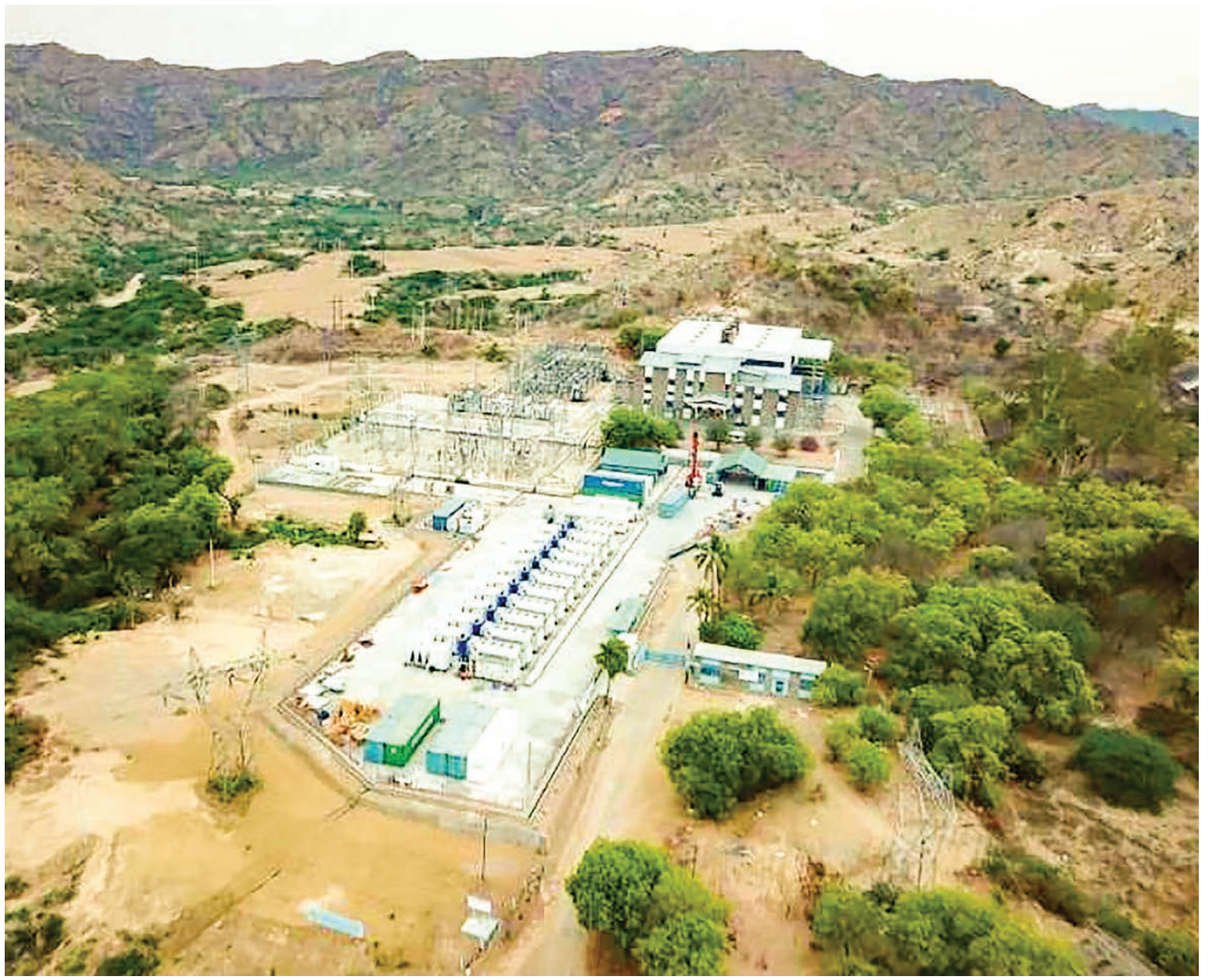
Kyun Chaung power plant.
