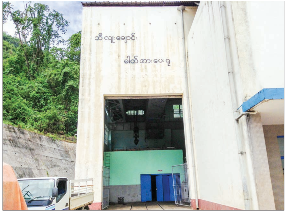
Biluchaung Hydropower Station
