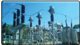
66/11 KV, 5 MVA transformer installation at Sittwe substation
