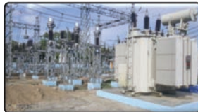
66/11 KV, 5 MVA transformer installation at Sittwe substation
