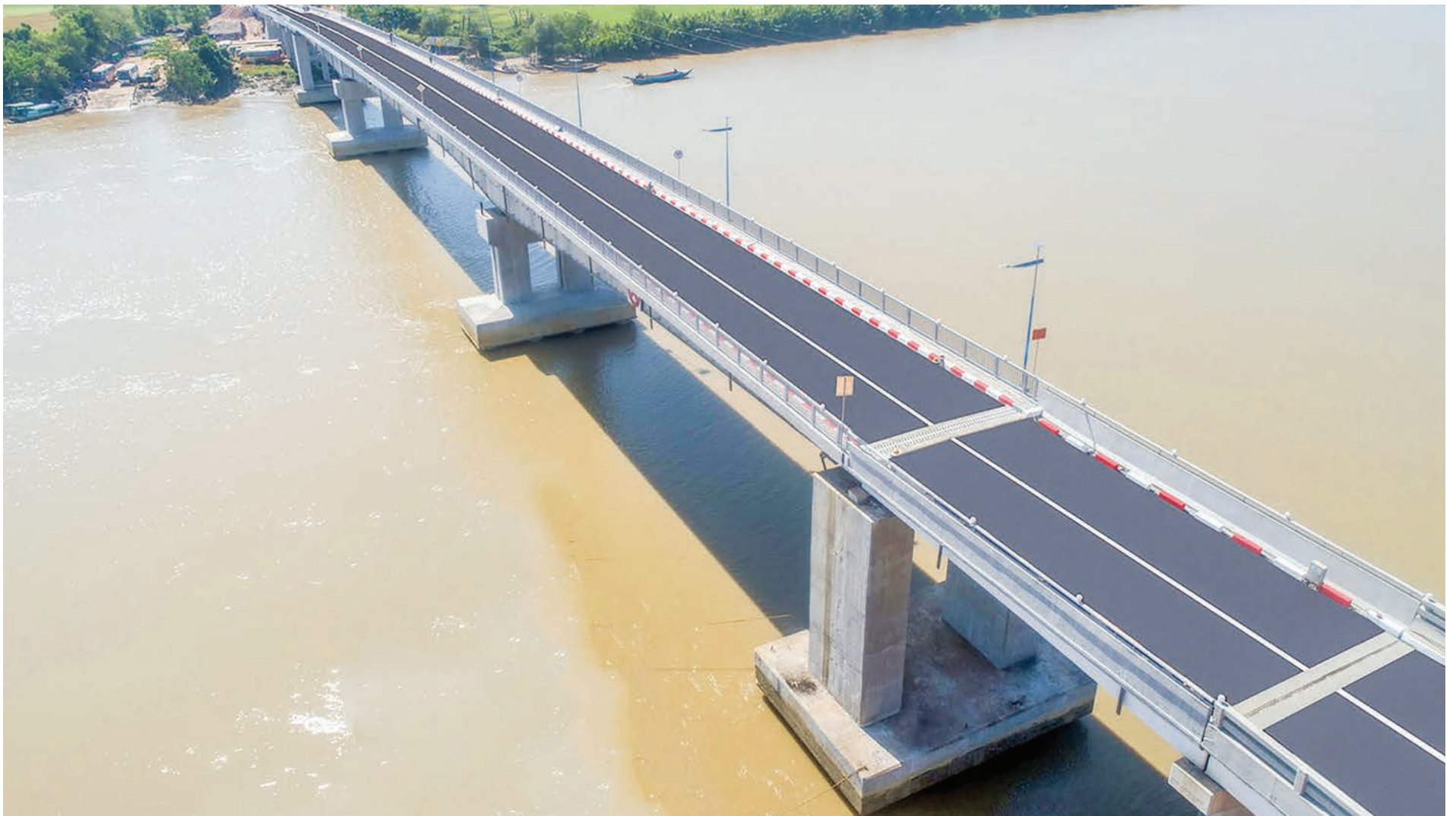
The Labutta (Pinlal Lay) Bridge was commissioned into service by State Counsellor Daw Aung San Suu Kyi in late December last year. PHOTO: MNA
