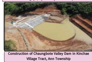
Construction of Chaungbote Valley Dam in Kinchae Village Tract, Ann Township
