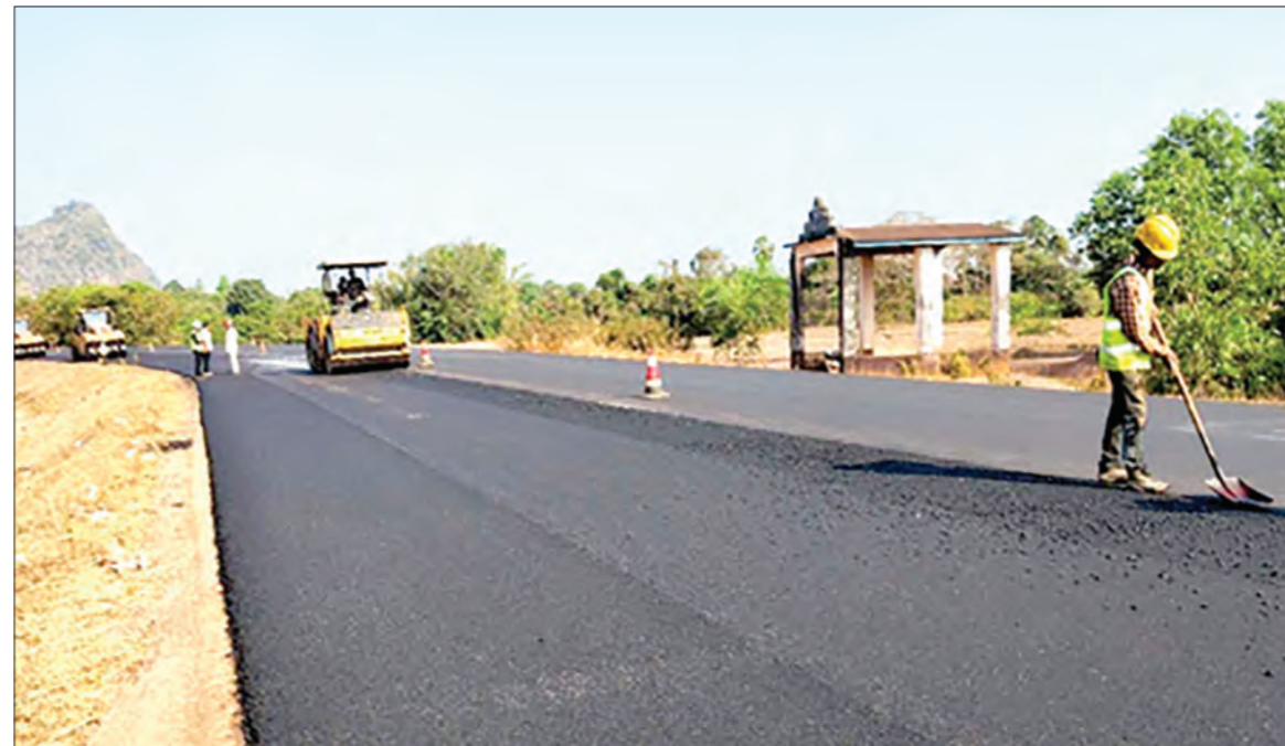
Eindu-Kawkareik Road is being upgraded on 5 Nov 2019.
