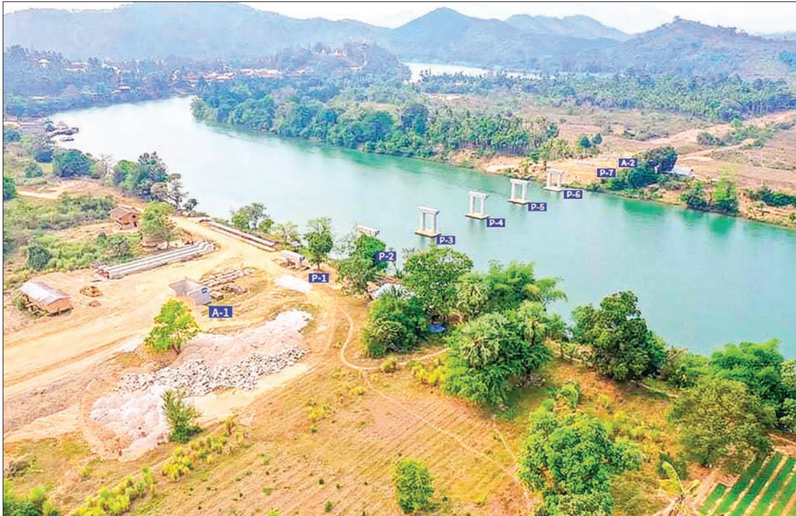
The 784.44 feet long Bawdikan Bridge seen under construction in Taninthayi Region.
