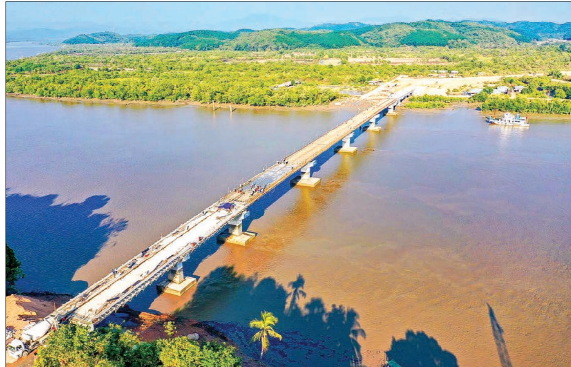
The 1287 feet long Thamoklutlut Bridge, seen under construction in Taninthayi Region.
