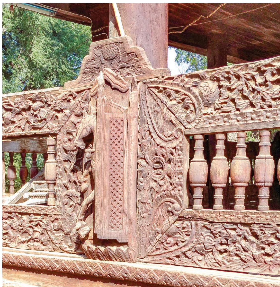
Sculptural works of First Three-storey Monastery
