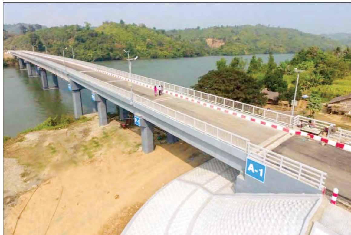
Darlat Creek Bridge on the Minbu-An-Sittway Road completed in the 2018-2019 financial year.
