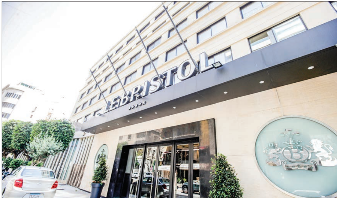
This picture taken on April 18, 2020 shows a view of the exterior of the five-star "Le Bristol" in the Hamra district of the Lebanese capital Beirut, which was forced to close for the first time since its opening in 1951 due to the worst financial crunch since the 1975-1990 civil war, now made more acute by a nationwide lockdown since mid-March because of the COVID-19 coronavirus pandemic. PHOTO: AFP
