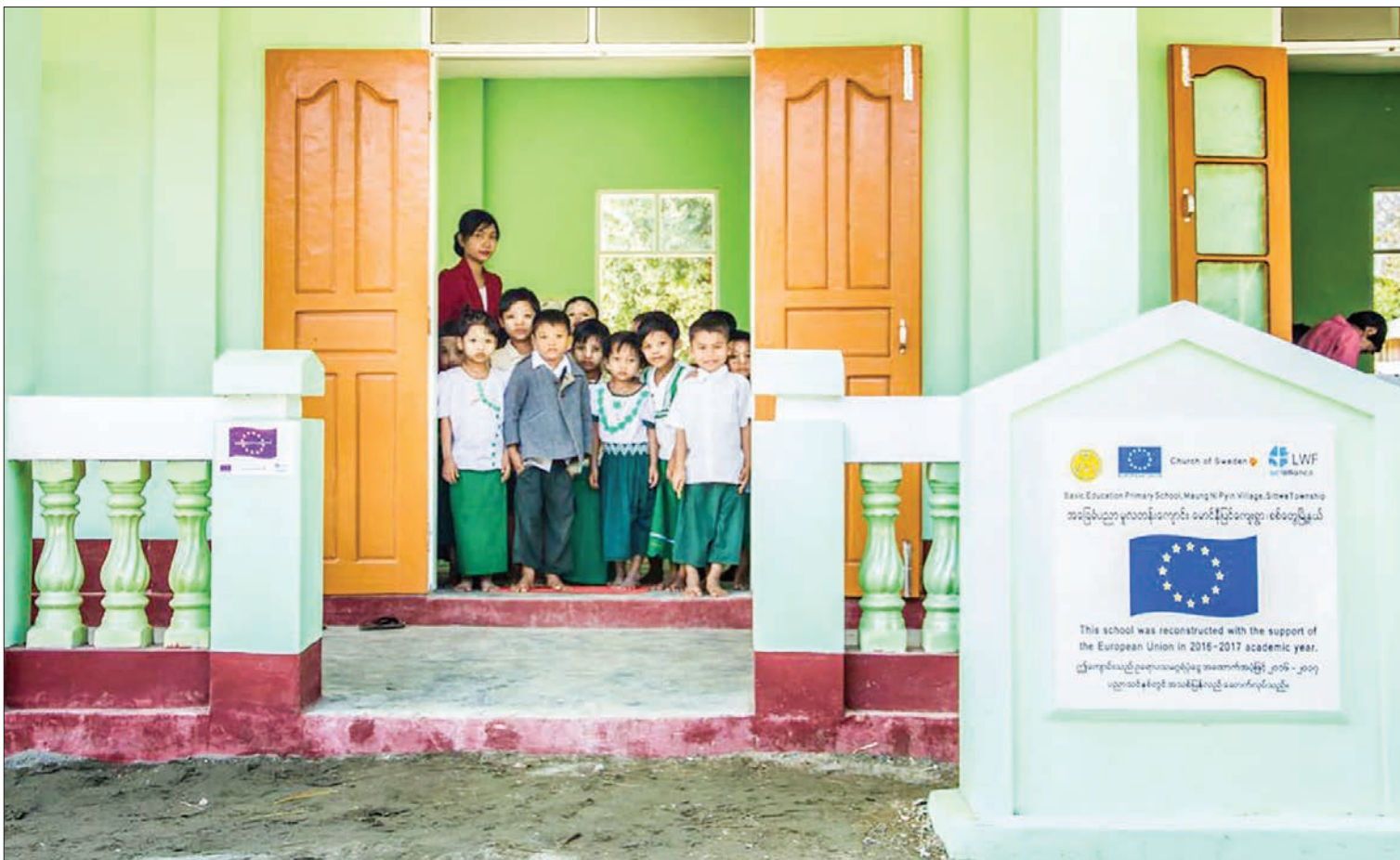
Reconstructed primary school in Rakhine State, financed by the EU. PHOTO: SUPPLIED
