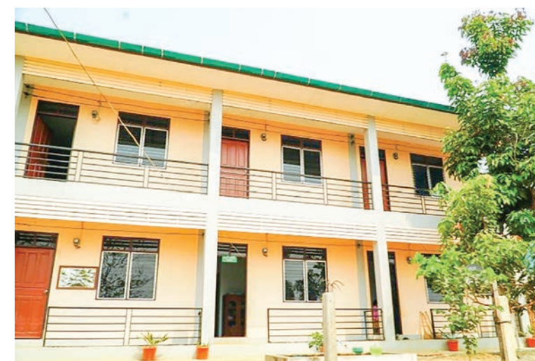
The two-storey staff housing of Basic Education Primary School (Kyaing Lat).
