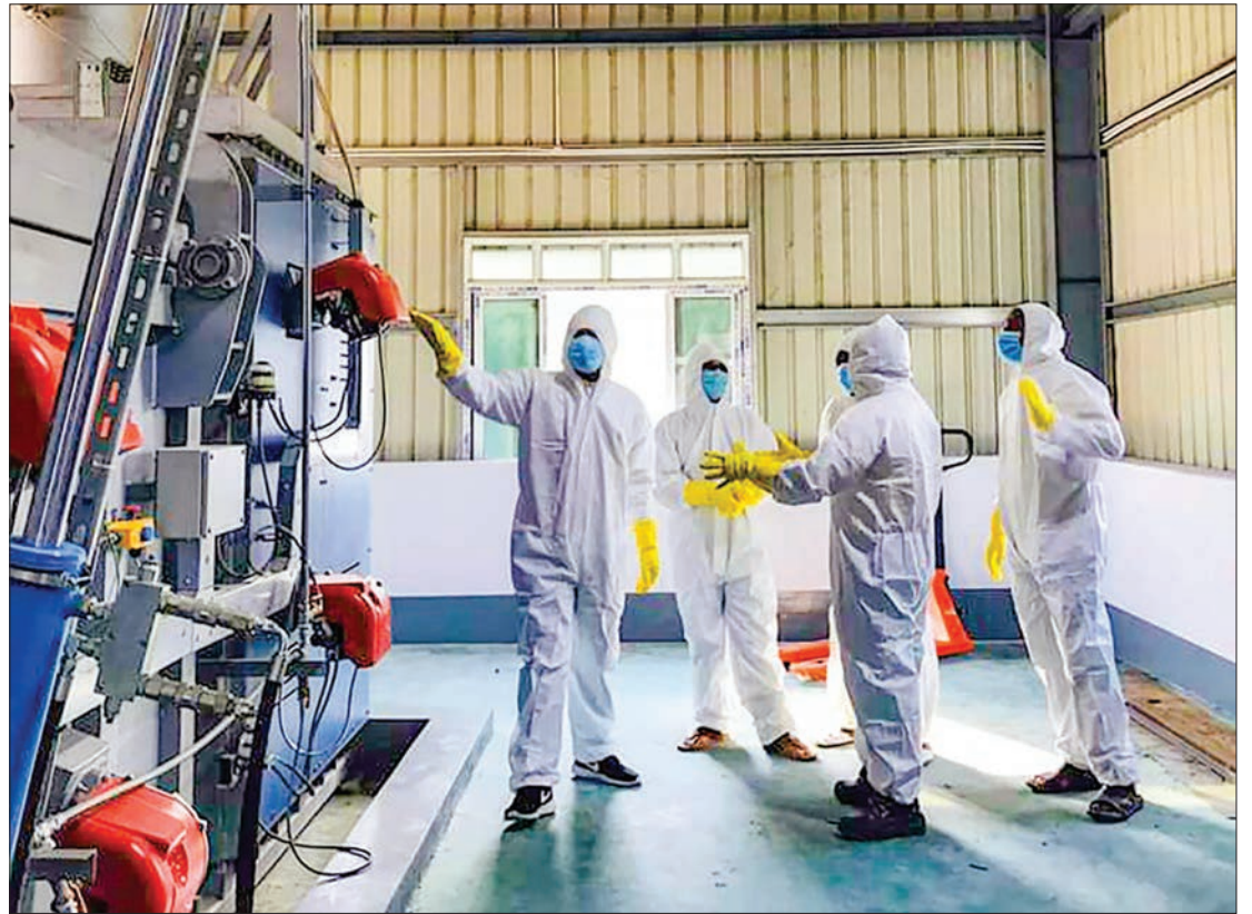
Staff operate the incinerator to burn the wastes. PHOTO: AUNG MYINT MAW
