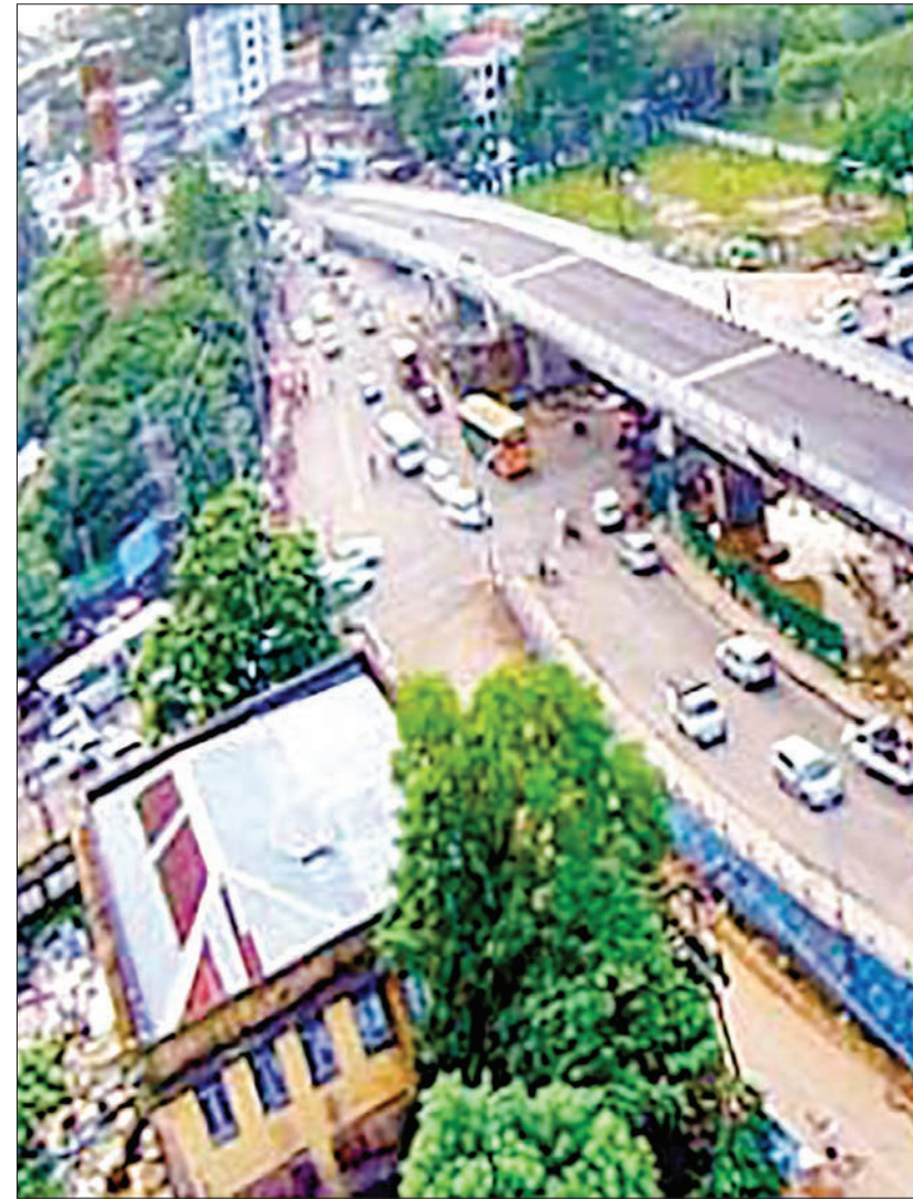
The photo shows Bayintnaung overpass at the junction of Bayintnaung. PHOTO: SHWE OO WAI
