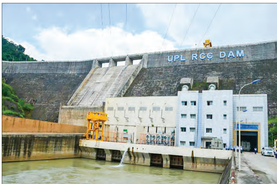
Upper Paunglaung Hydropower Plant.
