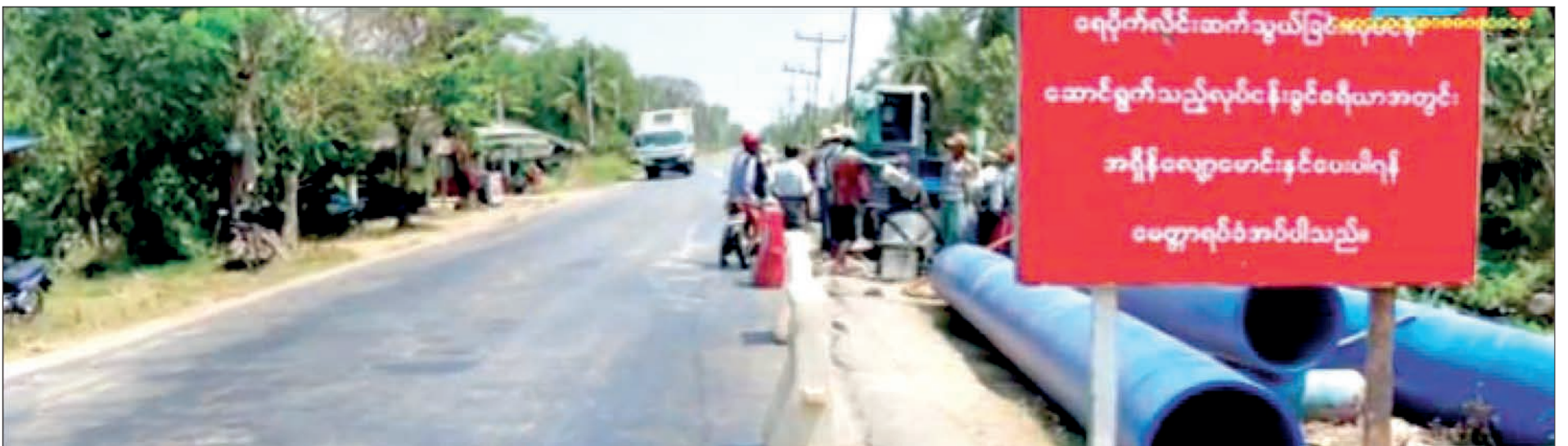
Municipal workers are in process of connecting water pipelines.
