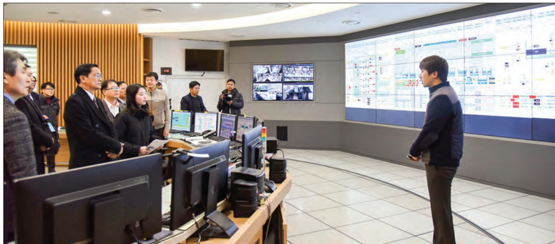
Vice President U Henry Van Thio observes the water distribution control room at Seoul Waterworks Authority in Seoul, the Republic of Korea yesterday. PHOTO: MNA
