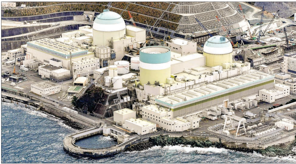
File photo taken Jan. 13, 2020, shows (from L) Nos. 3, 1 and 2 reactors of the Ikata nuclear power plant in Ehime Prefecture, western Japan. The Hiroshima High Court on Jan. 17 ordered its operator Shikoku Electric Power Co. to suspend the No. 3 reactor. PHOTO: KYODO NEWS
