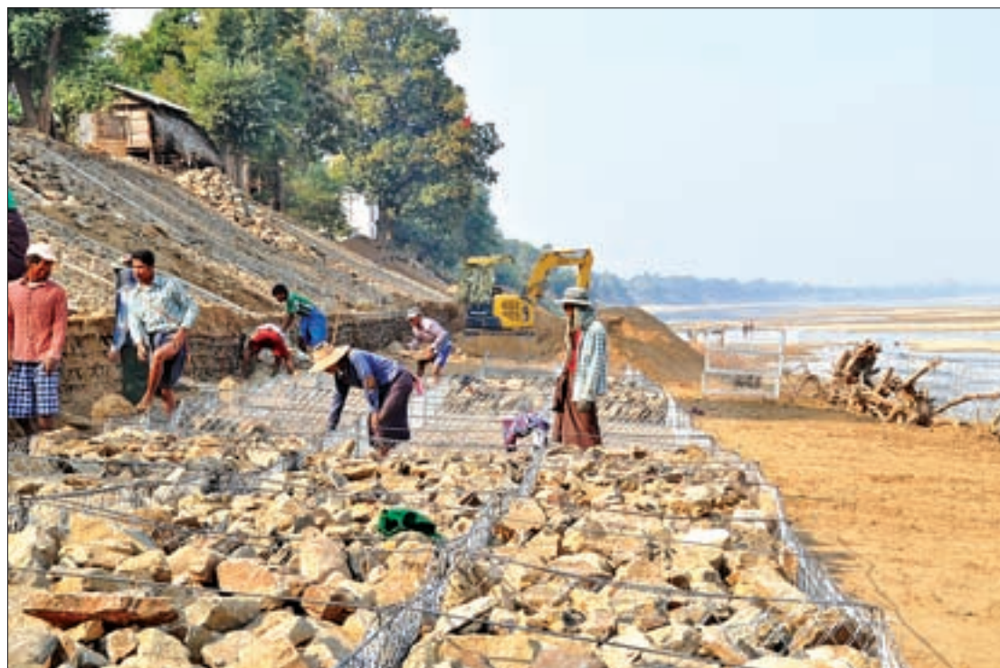
Workers lay stones at the bank of Ayeyawady River in Mandalay to prevent erosion. PHOTO: ATK
