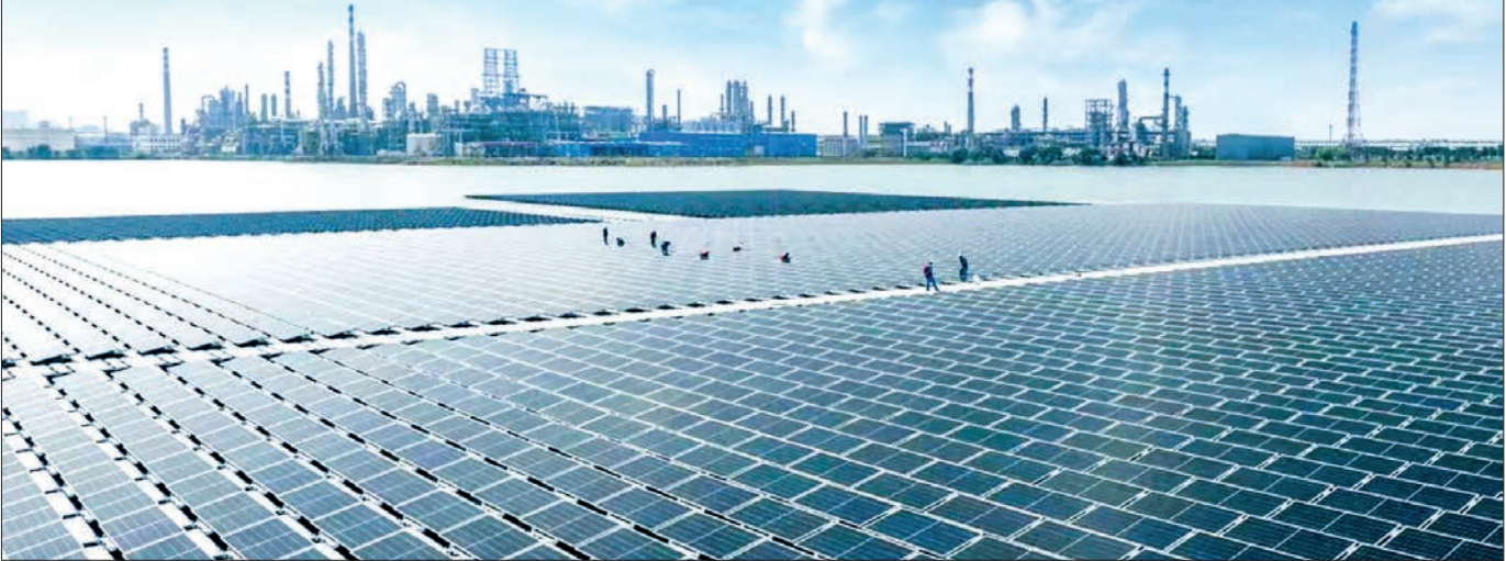
The 7.5 MW facility is Sinopec’s largest floating PV system to date, integrating an existing pile-based floating plant. It is located in a sea-connected area and is designed to be fully operational in a seawater environment. PHOTO: SINOPEC
