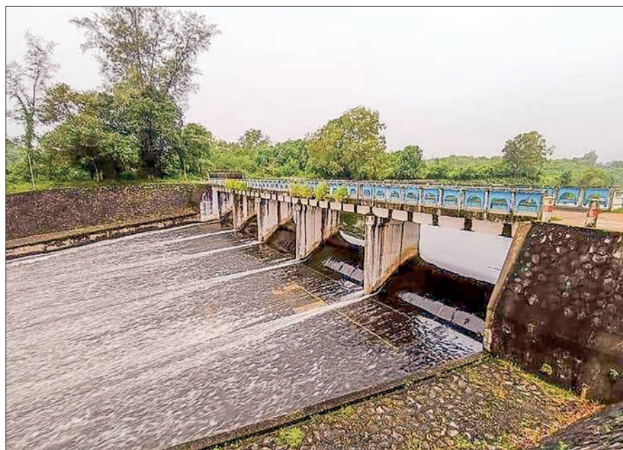
This photo depicts the conditions of the Ngamoeyeik Dam on 14 September 2024.
