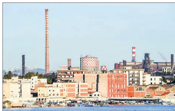
The steelworks date from the 1960s and have been dogged by battles over their killer emissions. PHOTO: ANDREAS SOLARO/AFP
