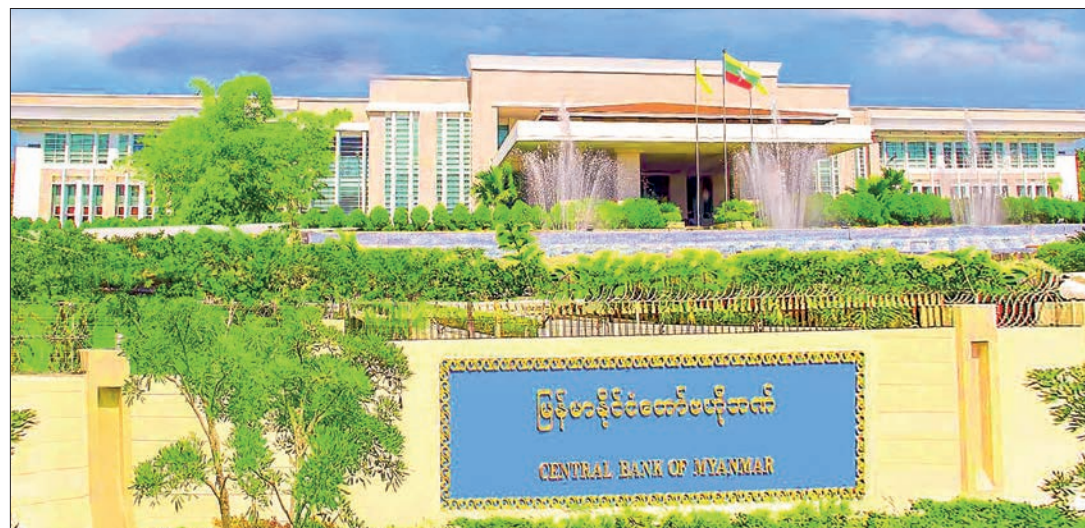
A glimpse of the general view of the Central Bank of Myanmar (CBM) in Nay Pyi Taw.
