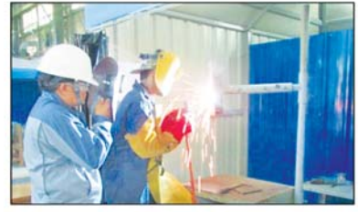
MIG/MAG (Gas Welding)
