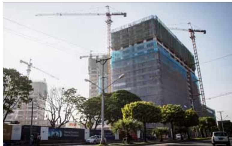
Construction work continues at the HAGL site. Photo: Zarni Phyto
