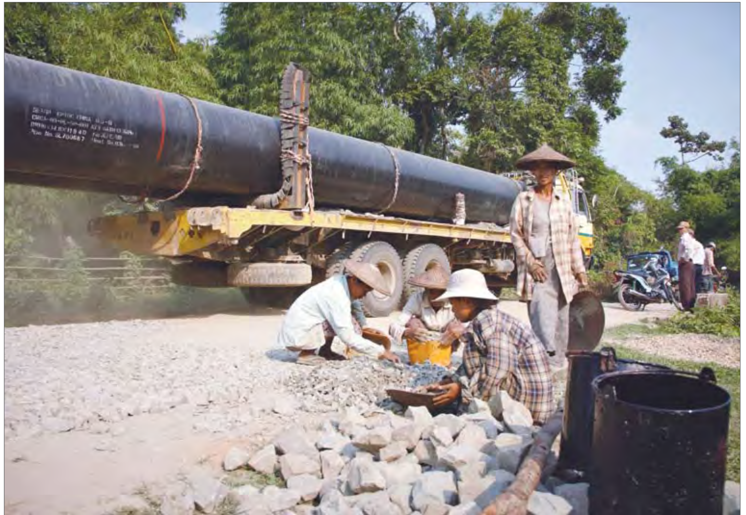
Local residents repair roads while a truck carries big gas pipes near Kyaukphyu in Rakhine State last May. PIC: JULIET SHWE GAUNG
