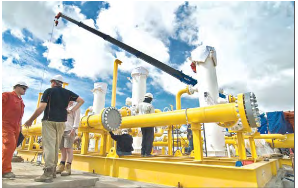
Technicians discuss onsite at a natural gas pipeline in southern Myanmar last year. PIC: KAUNG HTET
