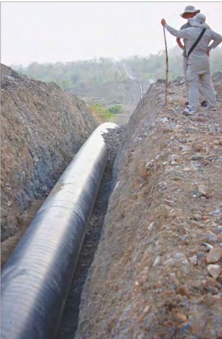
Two men chat near the Shwe gas pipeline in Kyaukphyu, Rakhine State.
