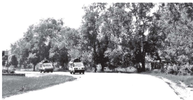
Photo shows Kyaikto-Thaton-Mawlamyine road section upgraded with advanced asphalt concrete.
