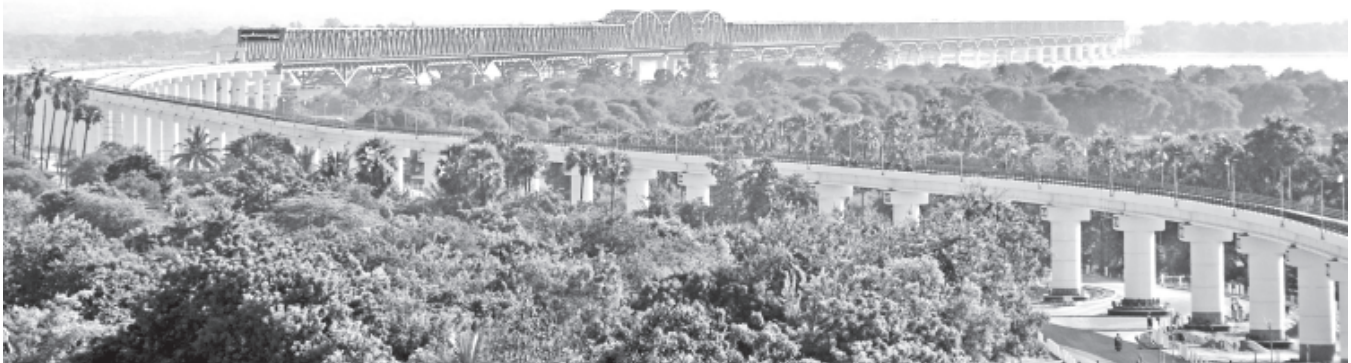
Photo shows Ayeyawady Bridge (Pakokku) in NyaungU Township to be commissioned into service soon.—MNA
