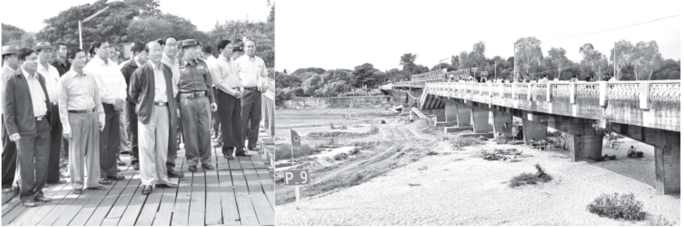
President U Thein Sein inspects construction of bailey bridge across Shwe Creek and site chosen for construction of new Shwe Creek Bridge.—MNA
