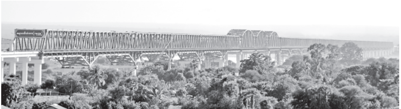
Photo shows progress in construction of Ayeyawady Bridge (Pakokku).—MNA
