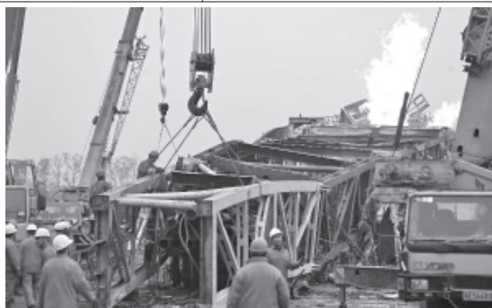
Rescuers clear up the fire scene at the Qionglai-1 gas well of China National Petroleum Corporation (CNPC), China's biggest oil and gas producer, in Dayi County, Chengdu, capital of southwest China's Sichuan Province, on 22 Dec, 2011. One person is missing and four others are hospitalized after the gas well exploded during a nitrogen drilling operation conducted here early Thursday morning. At present, the fire has been put under control and no toxic hydrogen sulfide gas was found in the gas leakage after the blast, said CNPC.—XINHUA
