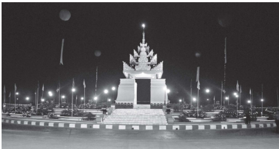
Photo shows Taguntaing Roundabout in Saga-in-TadaU-Taguntaing road section.—MNA
