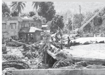
Workers survey a destroyed bridge in Iligan City, southern island of Mindanao, as the death toll from flash floods in the southern Philippines climbs above 1,000.—INTERNET
