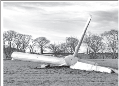
A wind turbine near Coldingham, Scotland, lays on its side after hurricane-force winds blew it down.
