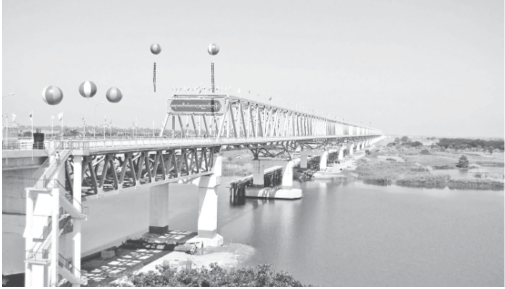
Photo shows already-opened Ayeyawady Bridge (Nyaungdon).—MNA
