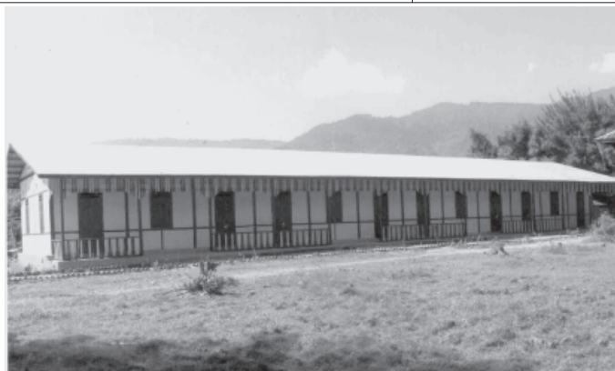
NEW SCHOOL BUILDING: Photo shows new post-primary school building, 120 feet by 30 feet, built in 2011-2012 fiscal year at a cost of K 19 million by State and K 13 million by local people in Ohnsansai Village of Mohnyin Township.—NLM-001
