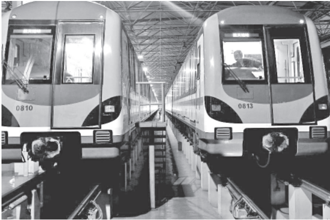
A technician checks the safety condition of a subway train at a base of metro line 8 at late night in Shanghai, east China, on 8 Nov, 2011. Eleven metro lines in Shanghai cover a total length of more than 425 kilometres. Technicians scattered in 18 metro bases, checking and repairing 370 subway trains. Usually, the technicians have to work all night long in order to ensure the trains run safely.—XINHUA
