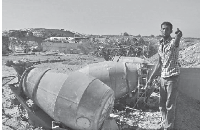
A Palestinian worker looks over a factory damaged in Israeli air strike on an adjacent site in Khan-Younis, southern Gaza Strip on 9 Nov, 2011. Israeli war jets carried out an air strike early Wednesday on training site belongs to Palestinian militants in retaliation to firing homemade rockets into southern Israel.
