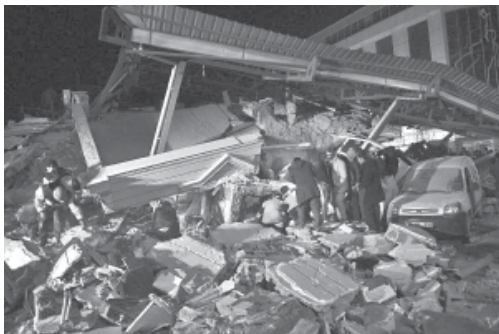
Rescue workers search for survivors at a collapsed building in Van, eastern Turkey, on 9 Nov, 2011. At least three people were killed when an earthquake hit Turkey's eastern Van Province on Wednesday and scores more were trapped beneath rubble of hotels and other buildings, state television reported.—XINHUA
