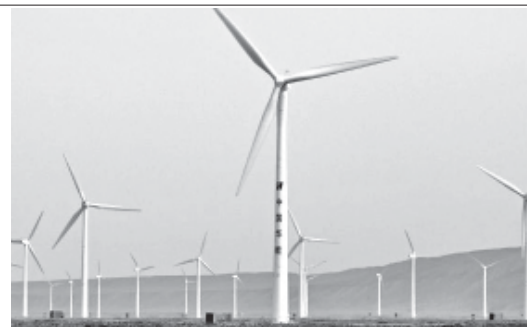
Photo shows the rows of windmills in the Gobi in Turpan, northwest China's Xinjiang Uygur Autonomous Region. The development of the pneumatic-electric power generating industry in Xinjiang has gained strong momentum since the country's strategy of development of the West, and the dense distribution of the windmills taking advantage of local affluent pneumatic energy become the new tourist attraction now.—XINHUA
