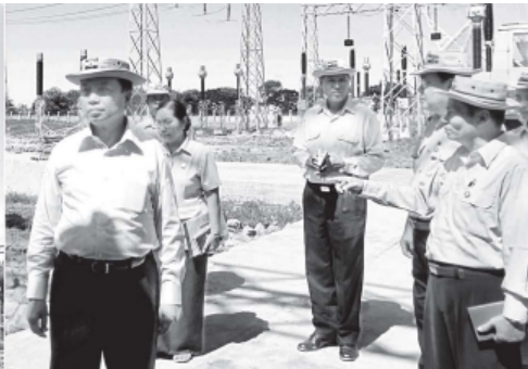
Union Minister for Electric Power No. 2 U Khin Maung Soe inspects 230 KV Myaukpyin main power station in Mandalay District.
