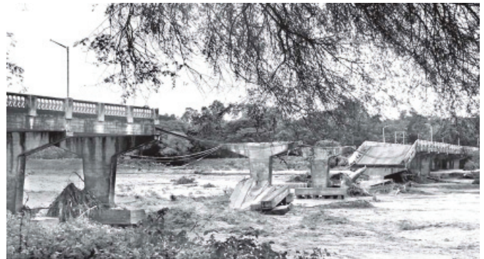
Photo shows Shwechaung Bridge on Pathein-Monywa road damaged by mountain torrent in heavy rains.
