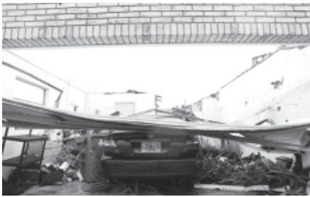
The garage door sits on a car in Sunrise, Fla on 19 Oct, 2011 after a possible tornado damaged more than two dozen homes in the area. Officials say a possible tornado left a 2 mile-long trail of damage in a suburban South Florida neighbourhood. Plantation Fire Battalion Chief Joel Gordon said Wednesday that the quarter-mile-wide debris trail has “all the classic signs” a tornado.—INTERNET
