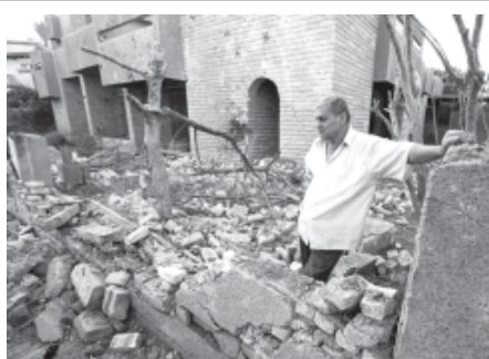
An Iraqi man inspects his damaged house after a bomb blast in Baghdad, Iraq, on 18 Oct, 2011. The Monday evening blast near a Baghdad liquor store killed at least seven people and injured another 18, Iraqi medical and police officials said.—INTERNET
