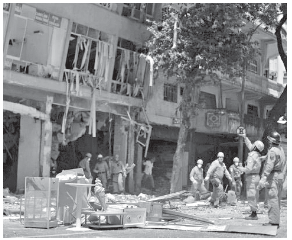
Firefighters work on debris of a restaurant in downtown Rio de Janeiro on 13 Oct, 2011. An explosion apparently caused by a gas leak ripped through a restaurant in downtown Rio de Janeiro early Thursday, killing at least three people and wounding at least 13, officials said.—INTERNET
