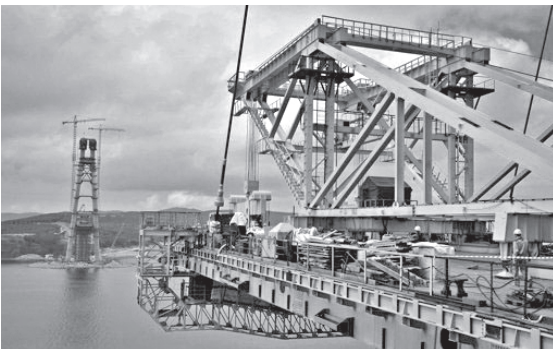
A bridge is being constructed to connect Russian Island to Vladivostok.—INTERNET
