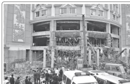
Photo shows the collapsed hotel gateway in Yifeng, east China's Jiangxi Province. —XINHUA
