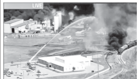
Video grab from CNN.com shows a major industrial fire at the Magnablend Inc chemical plant in Waxahachie, Texas, the United States, on 3 Oct, 2011.—XINHUA
