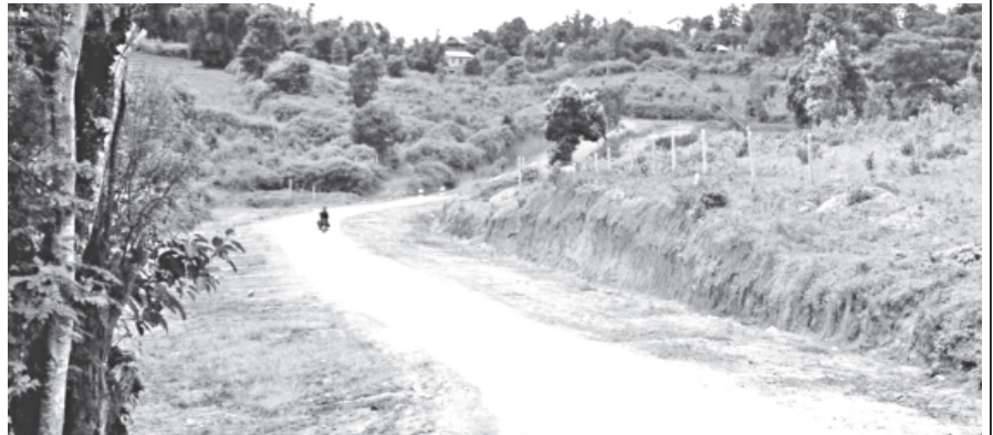
Photo shows a tarred road section on PyinOoLwin-Mogok road.
