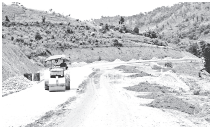
Rollers are ready for land preparation for tarmacking the road.
