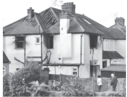
Neighbours view the remains of the house in Neasden, northwest London. A mother and five of her children were killed when a fire tore through the house, emergency services have said.—INTERNET
