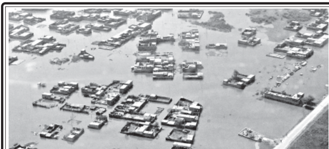
An aerial view shows destroyed houses in flooded area of Sanghar District of Pakistan's Sindh Province, 23 Sept, 2011. At least 369 people have died and 700,000 are living in refugee camps because of floods in southern Pakistan, the country's national disaster authority said.—XINHUA
