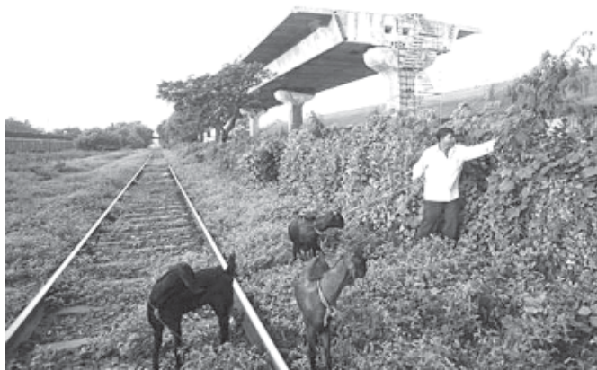
A man walks his goats near the construction site of new expressway in Mumbai on 20 Sept, 2011. Strapped for cash, New Delhi is pushing a model known as build-operate-transfer (BOT). Firms bid to build a road or a metro and operate it for a fixed period, collecting toll or ticket fares before handing it over to the government.—INTERNET
