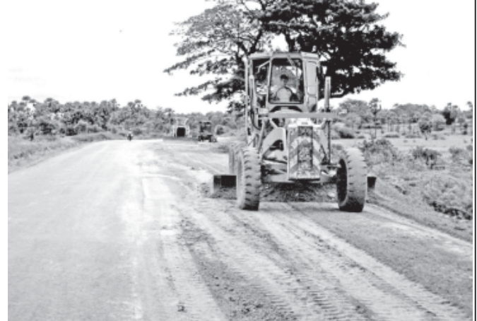
Heavy machinery at works to upgrade Meiktila-Kyaukpadaung-Bagan Road.
