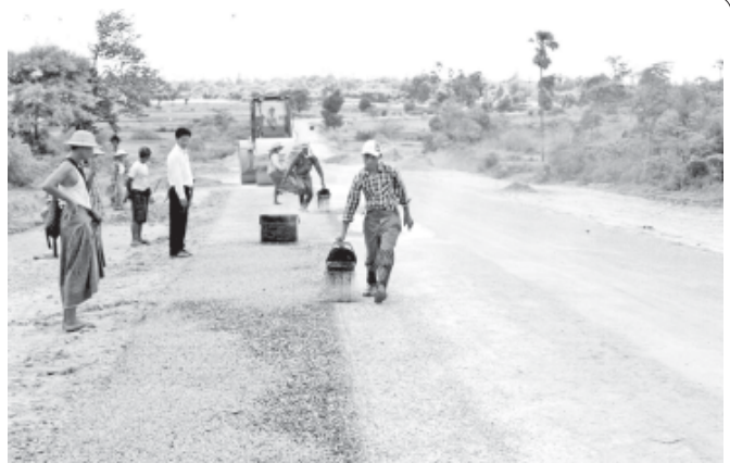
Workers of Myat Noe Thu Construction Company upgrading Meiktila-Kyaukpadaung-Bagan Road.
