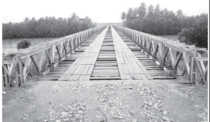
Auknatchaung Bridge on Bogale-Sathsan-Htawpaing-Amar Road in Bogale Township, Pyapon District.
