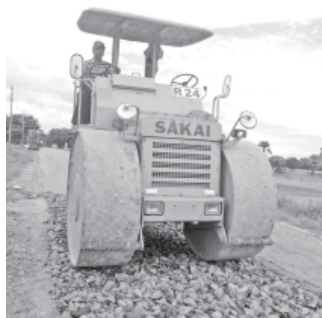
Heavy machineries engaging in roadwork of Hinthada-Hsongon-Myanaung road section.
