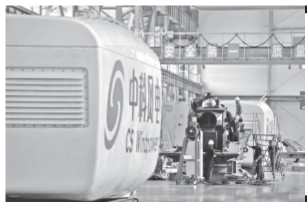
Technicians install wind turbines in a factory of CS Windpower Co, Ltd. in Tongliao City, north China's Inner Mongolia Autonomous Region, 2 Sept, 2011. INTERNET
