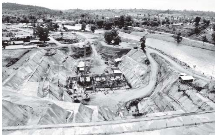
Photo shows progress in construction of Thaukyaykhat (2) Hydropower Project.
