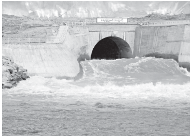
Photo shows water diversion tunnel of Thaukyaykhat (2) Hydropower Project.
