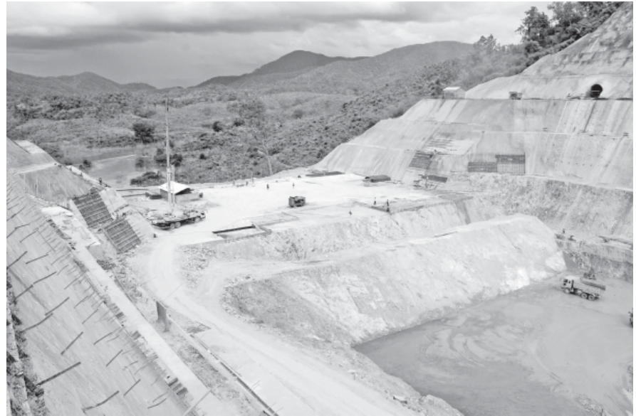
Progress in construction of spillway seen at Thaukyaykhat (2) Hydropower Project.
