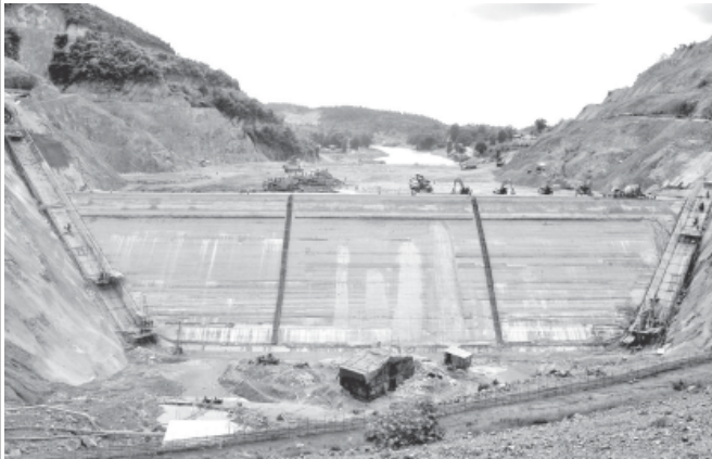
Photo shows construction of main embankment at Thaukyaykhat (2) Hydropower Project.
