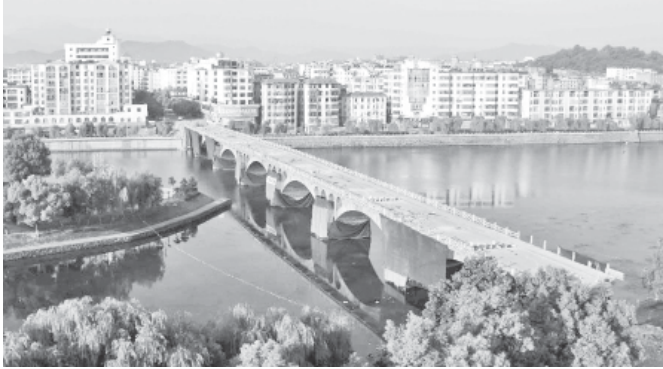
Photo taken on 20 Aug, 2011 shows the Yichun Bridge before demolition in Yichun City, east China's Jiangxi Province. The 284-meter-long bridge, built in 1970, will be replaced by a newly-built 1,760-meter-long one, which is scheduled to come on stream in June 2013.—XINHUA
