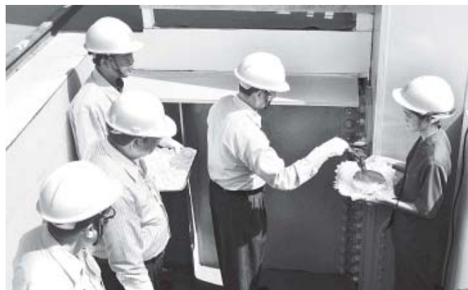
Union Minister for Construction U Khin Maung Myint fixing the final golden screw to Ayeyawady Bridge (Nyaungdon).
