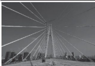
Photo taken on 18 Aug, 2011 shows the south main bay of the Erqi Yangtze River Bridge in Wuhan, capital of central China's Hubei Province. The two sections of the south main bay of the bridge were joined on Thursday. The 6,507-meter-long bridge with six lanes is expected to be put into operation in the end of 2011. XINHUA
