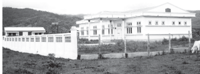
Photo shows 66/11KV 5MVA power station near Government Technological College in Mohnyin.—NLM 001
